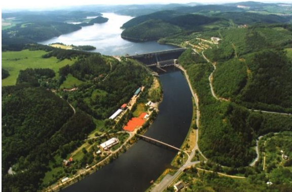
Figure 7 – Aerial view of the Orlik reservoir
