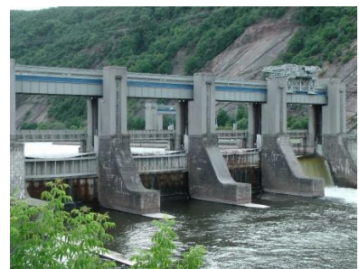
Figure 24 – Vrané Hydroelectric Power Plant
