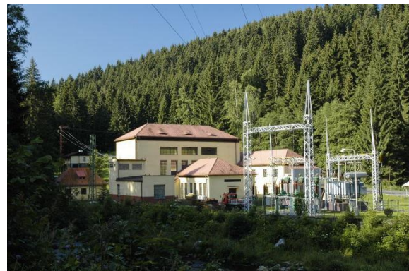
Figure 16 – New building of the Čeňkova pila Hydroelectric Power Plant
