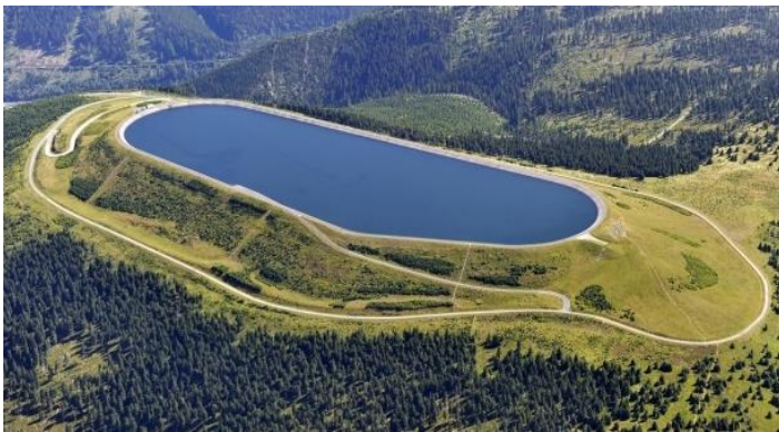
Figure 11 – Aerial view of the upper reservoir
