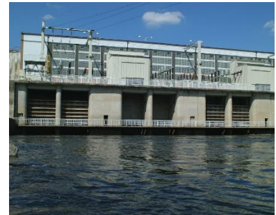
Figure 21 – Kamýk Hydroelectric Power Plant
