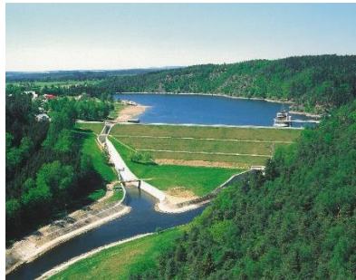
Figure 20 – Hracholusky Hydroelectric Power Plant
