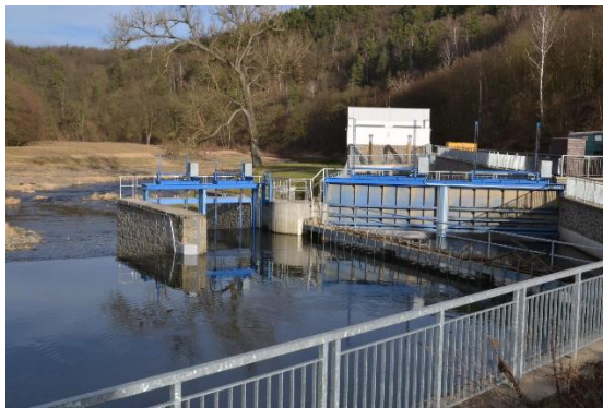
Figure 17 – Bukovec Hydroelectric Power Plant
