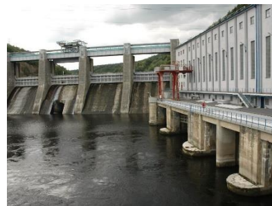
Figure 23 – Štěchovice II Hydroelectric Power Plant
