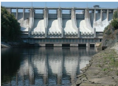
Figure 22 – Slapy Hydroelectric Power Plant
